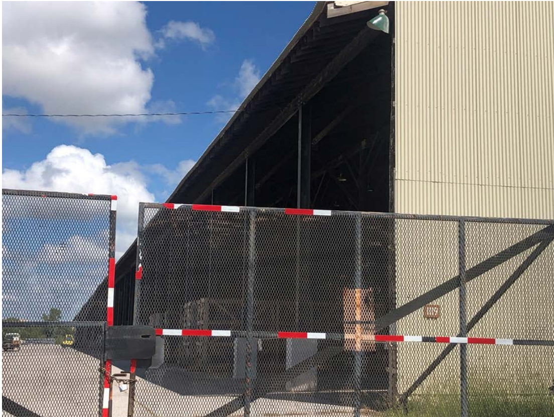
Figure 2-4. Example Pole Barn Building
